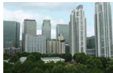
Indecon Court, London, United Kingdom – Decentralized System
